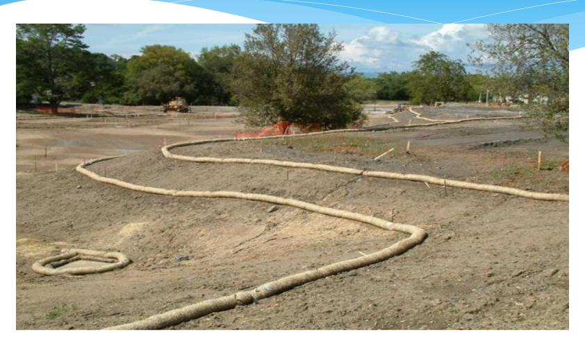
This is an example of Sediment and Erosion control at a bridge installation over a fish bearing stream utilizing jute mat and straw wattle.
