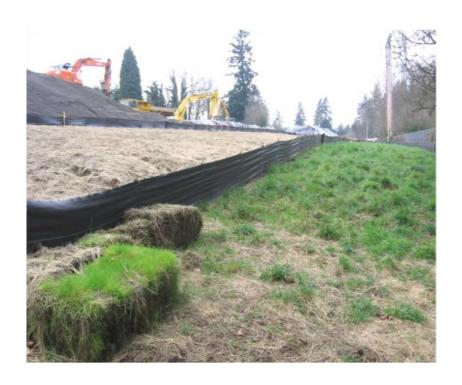
BMP C122. Erosion control nets and blankets are intended to prevent erosion and hold seed and mulch in place on steep slopes and in channels so that vegetation can become established. Jute mat shown. Usually biodegradable materials such as Jute, Coconut or Straw weave.
