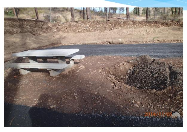
BMP C105. Construction entrances are stabilized to reduce the amount onto paved roads by vehicles or equipment by constructing a stabilized pad of quarry spalls at entrances to construction sites.
